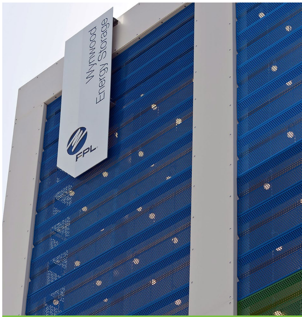
FPL Wynwood Energy Storage in Miami, Florida.
