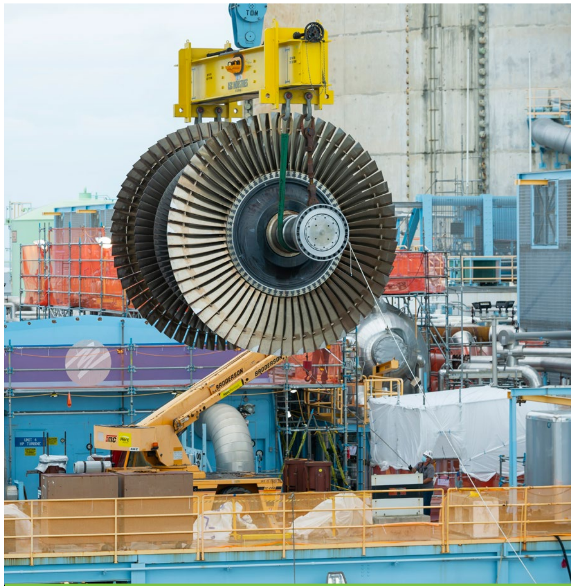
Crews lift a large rotor during a maintenance outage of Unit 4 at the Turkey Point Nuclear Power Plant near Homestead, Florida.
