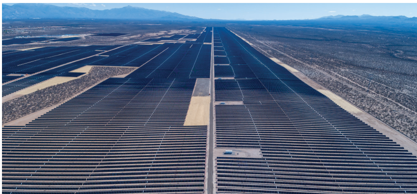
NextEra Energy Resources' Wilmut Energy Center in Arizona combines 100 MW of solar energy and 30 MW of battery energy storage.
